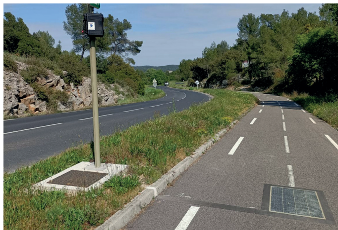
1 Wattway slab makes the bicycle counter autonomous
