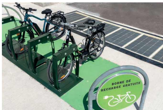
A 6-panels Wattway Pack enables the self-sufficiency of 4 bicycle charging stations
