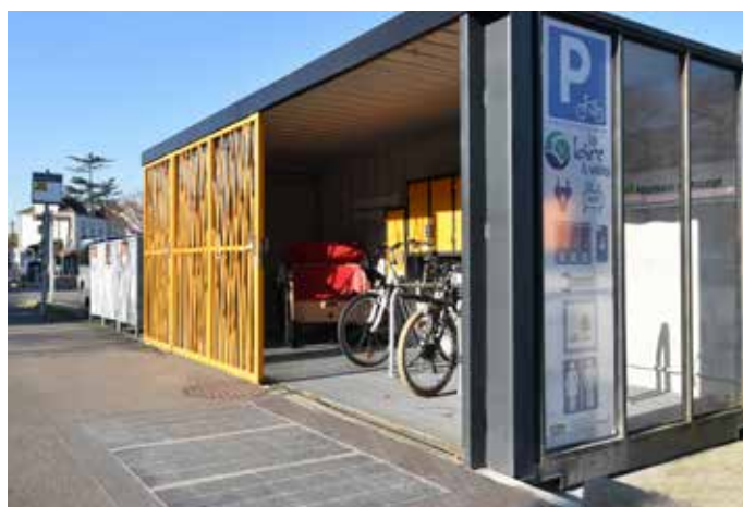
The Nielsen Concept Mobilités bicycle shelter is self-sufficient in energy thanks to Wattway Pack
