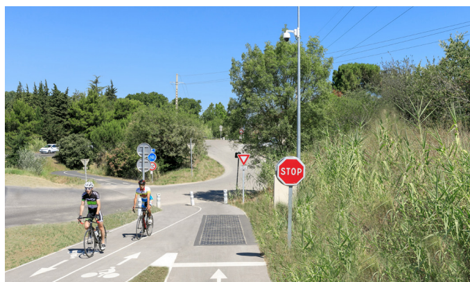
Montpellier, France – 12 panels power a surveillance camera.
